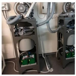
Example of use of wet suction system with a sedimenting amalgam separator
